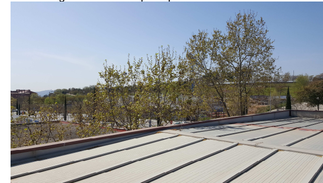
Vista carener coberta principal
