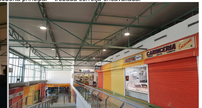
Vista general interior coberta principal
