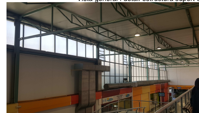
Vista general interior coberta principal
